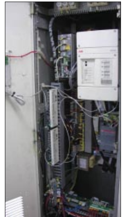
Port of Miami: the picture above shows the E-house drive module with ABB Tyrak L drive; the picture below shows it after upgrade to ABB DCR 600
